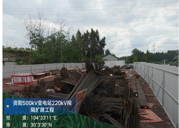
材料堆场区临时铺垫
