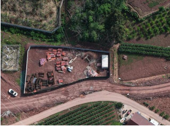
材料堆场区临时铺垫
