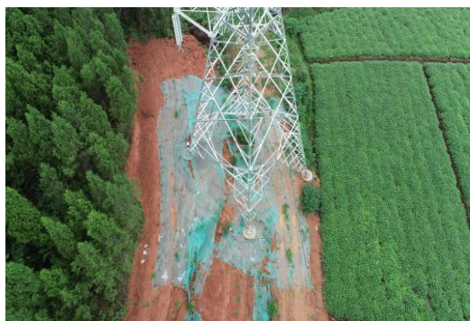
N20 临时苫盖
