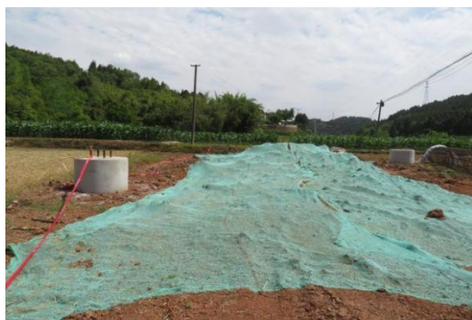
N19 临时苫盖
