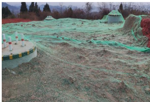
NA12 塔基临时苫盖
