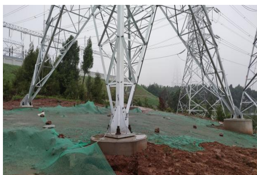
N1 临时苫盖
