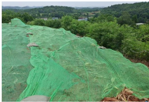
M12(N33)塔基临时苫盖
