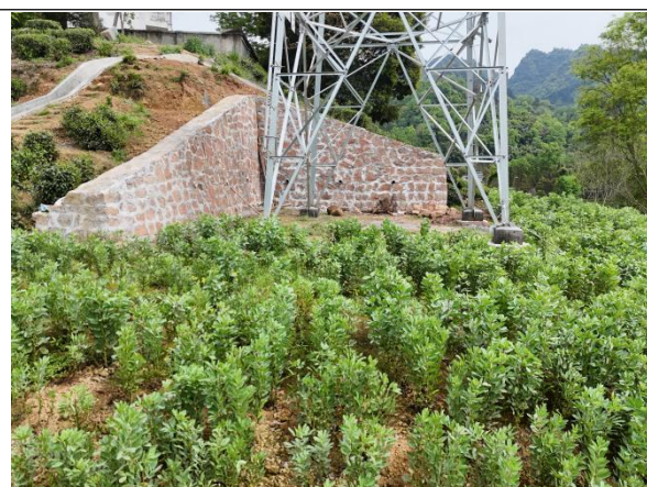
N57 塔基处堡坎及排水沟 (2026.2)
