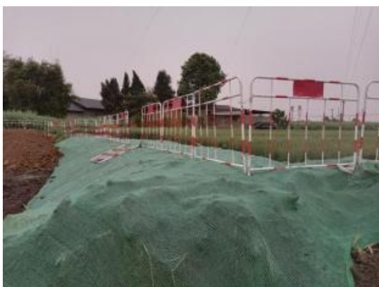
N379塔位临时遮盖
