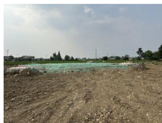
N359塔位临时遮盖
