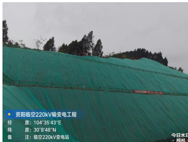
边坡临时苫盖
