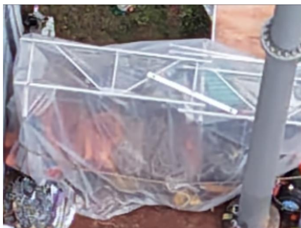
间隔扩建临时苫盖
