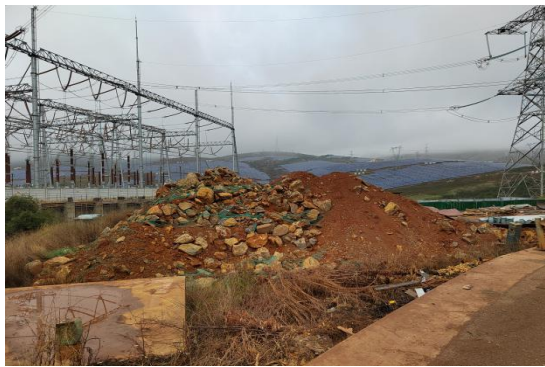
临时堆土临时苫盖
