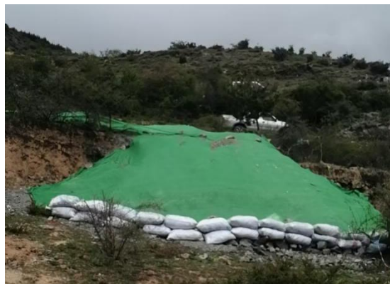
N18 塔基边坡土袋拦挡及临时苫盖
