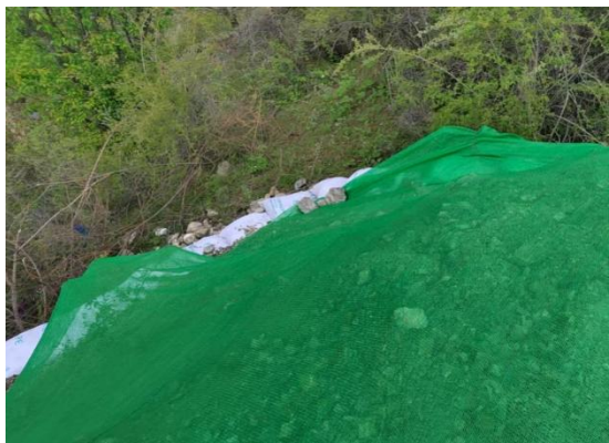
N5 塔基边坡土袋拦挡及临时苫盖
