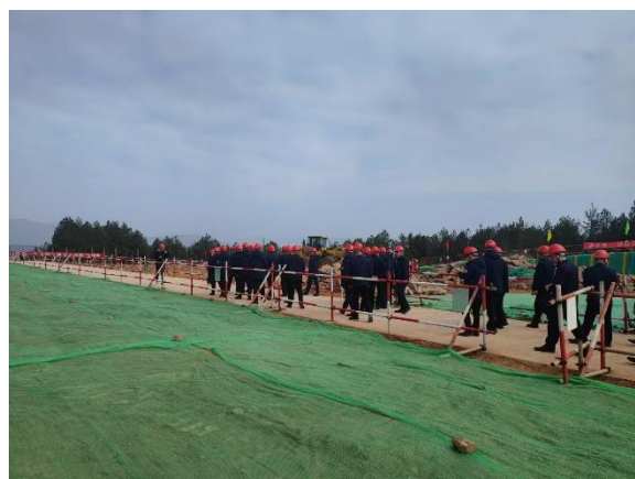
裸露地表临时苫盖
