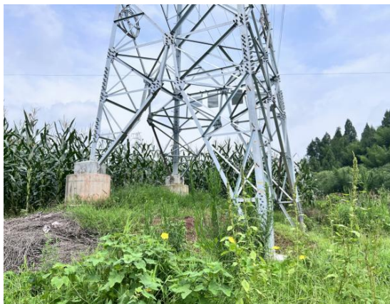
N20#塔植被恢复
