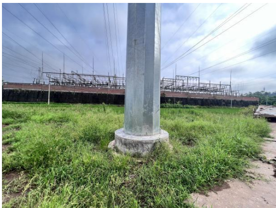
N1#塔植被恢复
