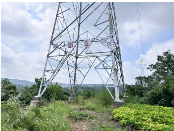
N16#塔植被恢复
