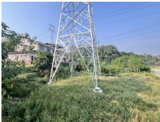
N2#塔植被恢复
