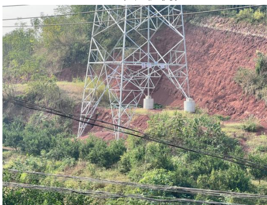
N22#塔植被恢复
