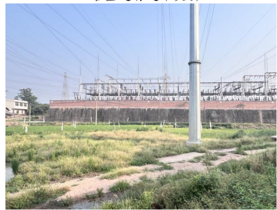
N1#塔基牵张场场地恢复现状
