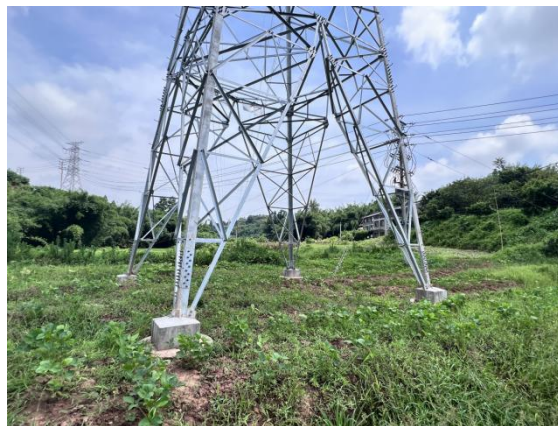
N21#塔植被恢复
