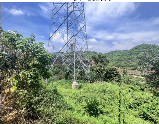
N26#塔植被恢复
