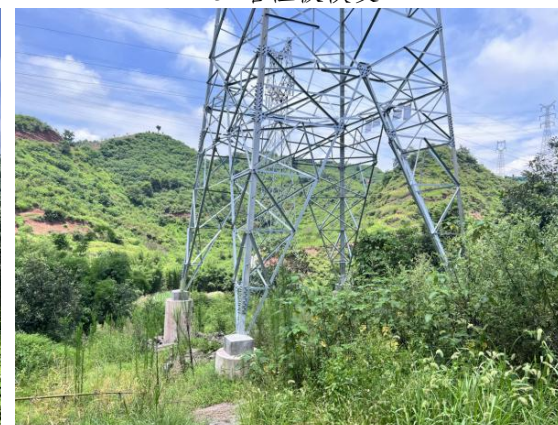
N27#塔植被恢复
