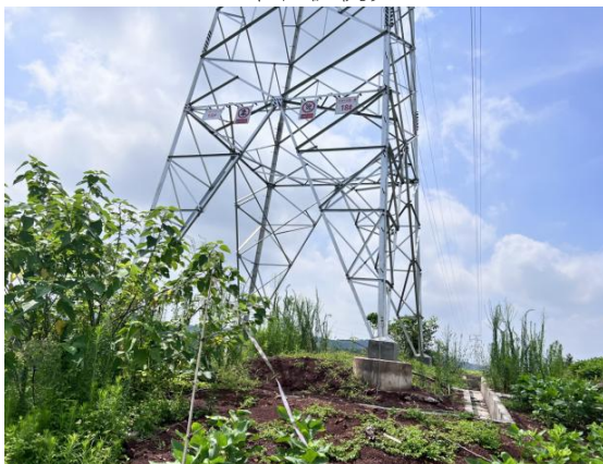
N17#塔植被恢复
