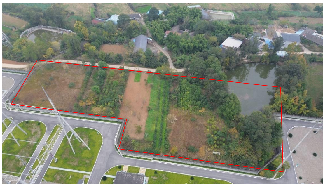
扩建区域航拍现状 2 (2023.11)
