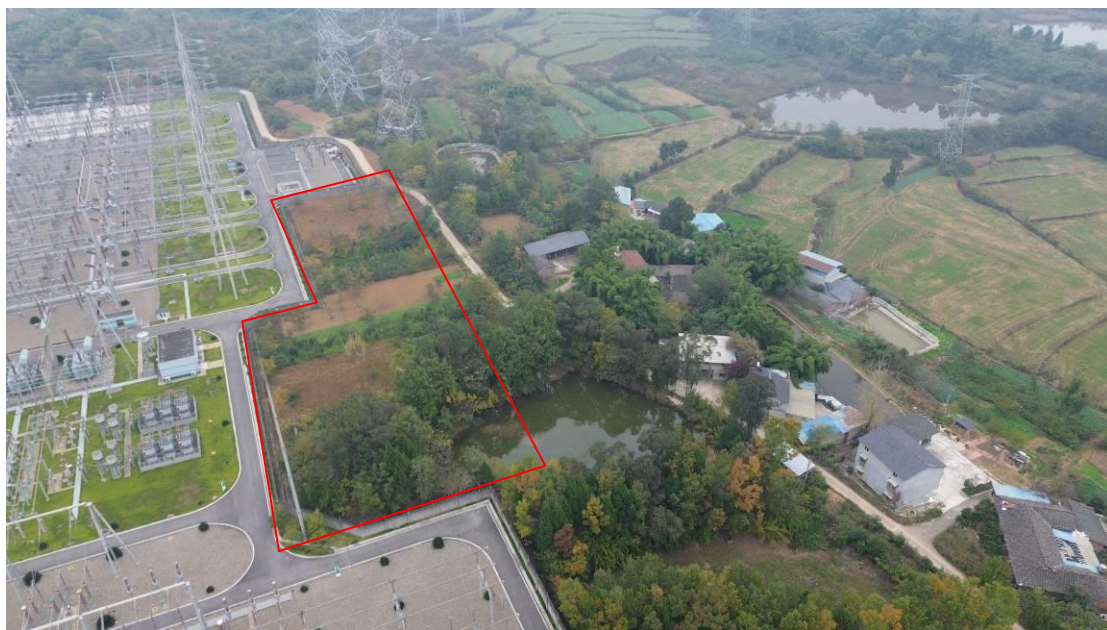
扩建区域航拍现状 1 (2023.11)
