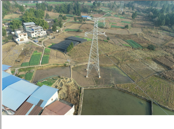
阆北-马鞍牵引站（N54）-导线展放后场地现状
