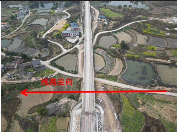
况井线、况江支线电缆排管穿越渝昆高铁 (2023.3)
