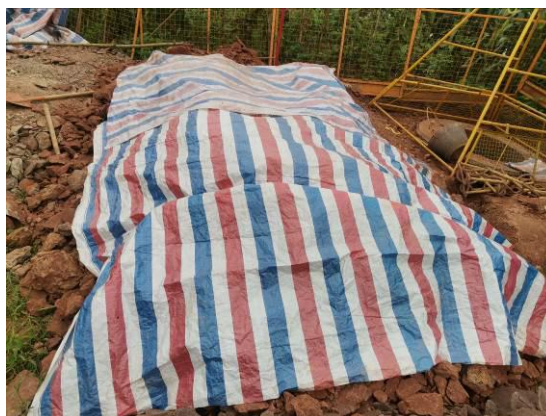
泸州东~林庄 N37 临时苫盖
