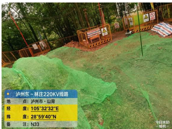
泸州东~林庄 N33 临时苫盖
