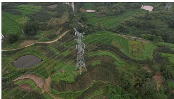
泸州东~泰安 N21 塔基施工临时占地复耕
