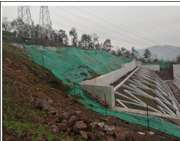
边坡治理区临时苫盖
