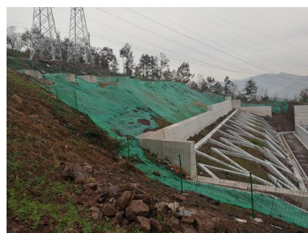
边坡治理区临时苫盖
