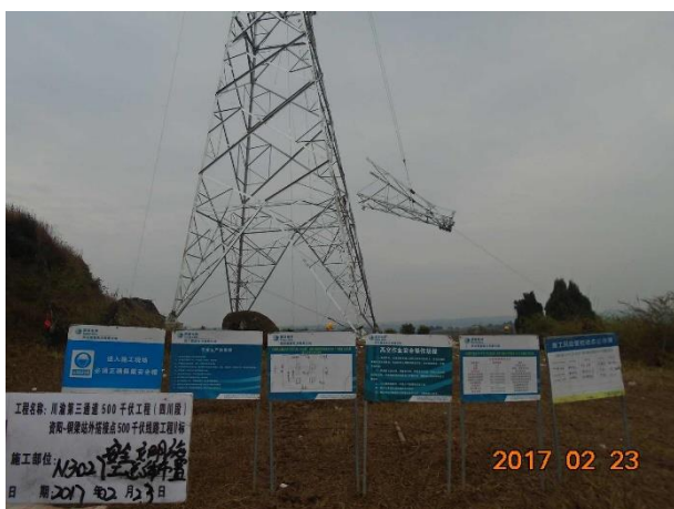
N3041塔基施工面貌 (2017.2)
