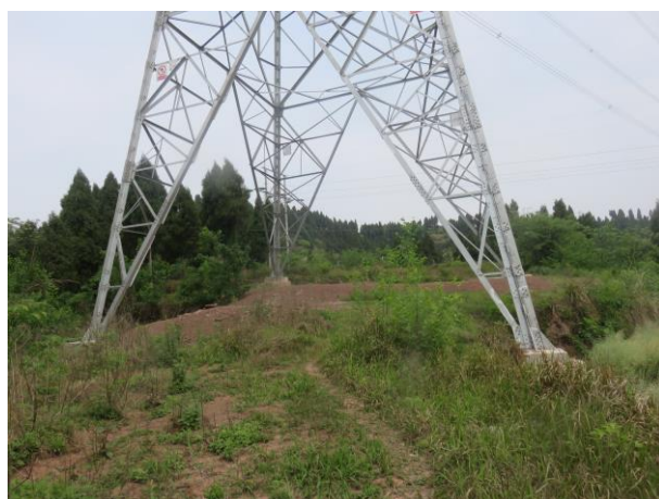
N3041塔基植被恢复 (2018.4)
