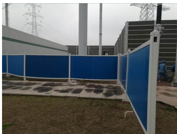
资阳变扩建区施工临时拦挡 (2017.3)
