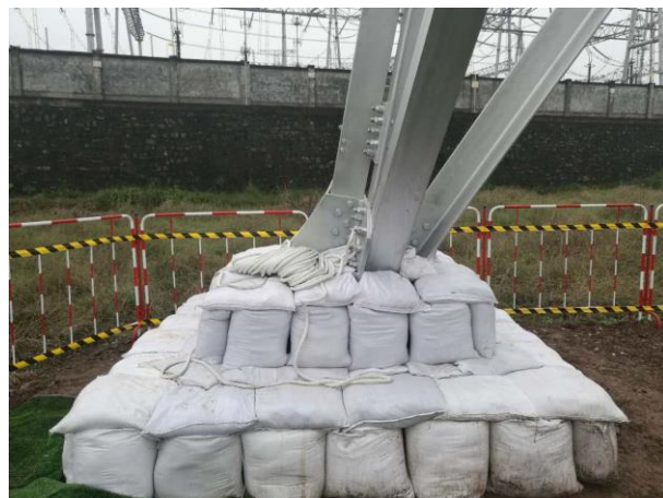
塔基临时拦挡 (2017.2)
