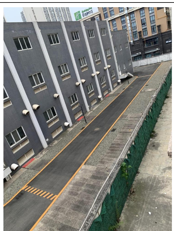
变电站内布置
