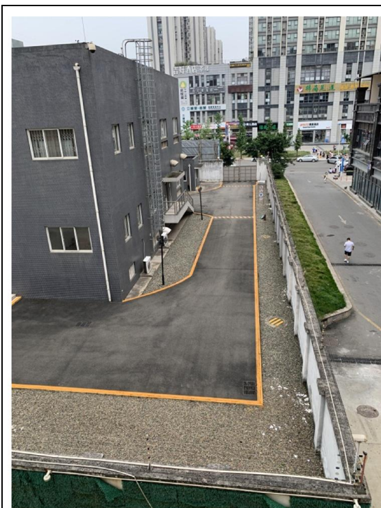
变电站内布置
