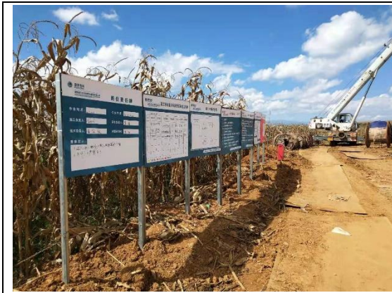
N20 牵张场钢板铺垫
