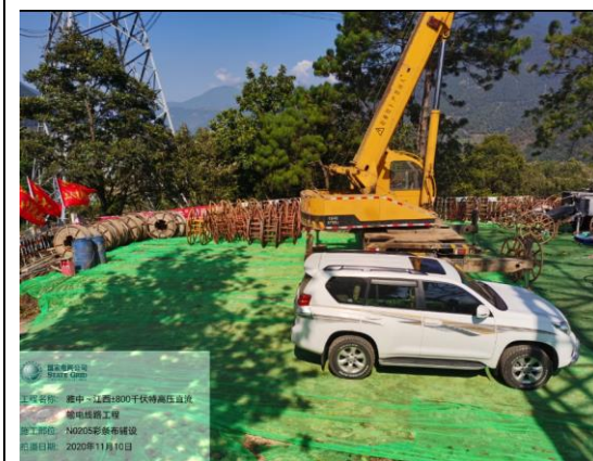
N0205 牵张场防尘网铺垫
