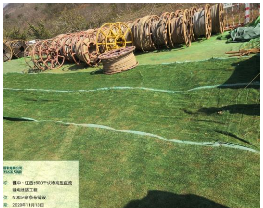
N0054 牵张场防尘网铺垫
